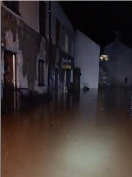
Figure 6: Flooding on Mill Street (Source: Real Fans of Ruthin Facebook page)
