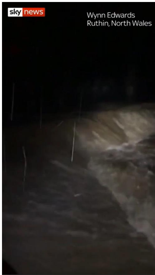
Figure 8: Overtopping of the Cae Ddol embankment (source: Sky News 3 )
