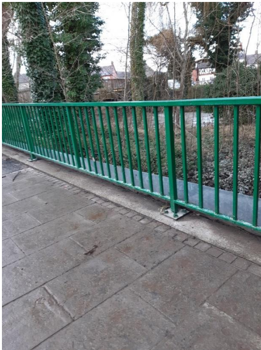
Figure 9: Steel plate flood wall along Clwyd Street (source: NRW staff)
