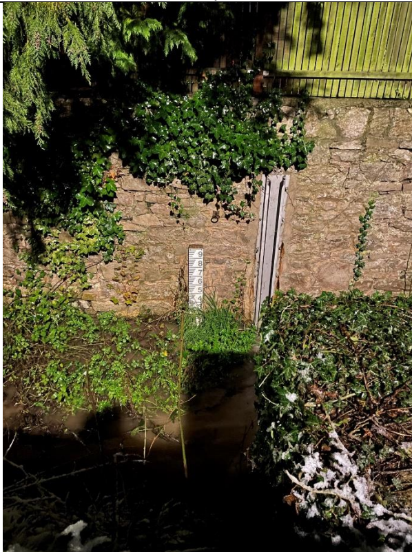
Llanfwrog open channel water level
