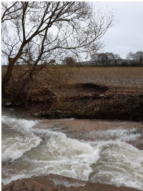
Image 3. Area of scour on right bank adjacent to weir.
