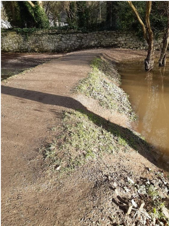
Figure 4: Cae Ddol embankment near skatepark (source: NRW staff)
