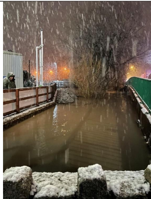
Outfall view – BT garage to left, road bridge to right
